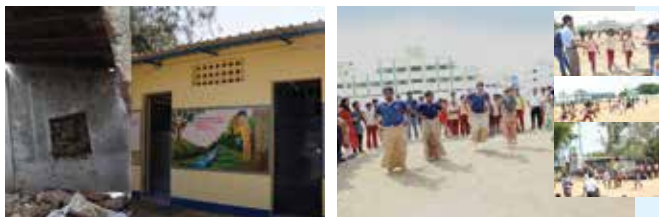
Re-constructing of toilet facilities
