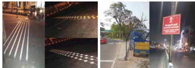
Placement of rumble strips and cat eyes in accident prone zone
