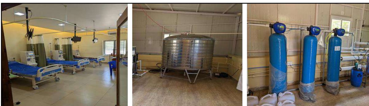
Figure 5 Dialysis cot, Effluent treatment plant and Automatic -RO Plant 1000/PH/ Lit Capacity
